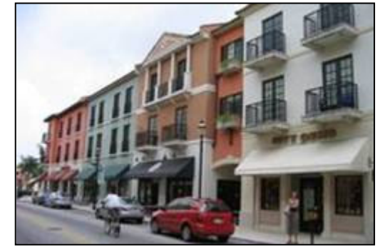
FIGURE 4.6 Façade variation and attention to detail, such as balconies and awnings, help to break up the mass of a large building
