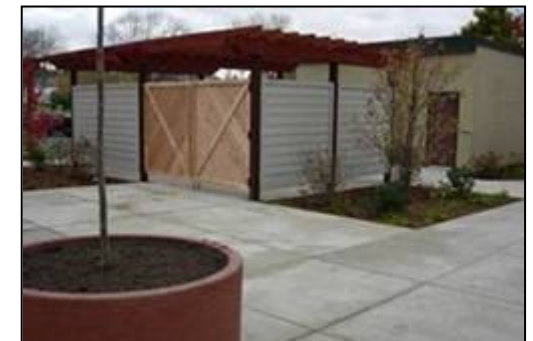
FIGURE 4.8 Simple structure to hide trash bins can make a large aesthetic difference
