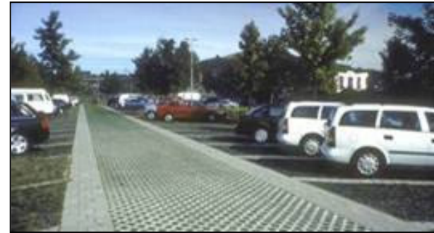
FIGURE 4.14 Permeable surface parking lot that incorporates stormwater
